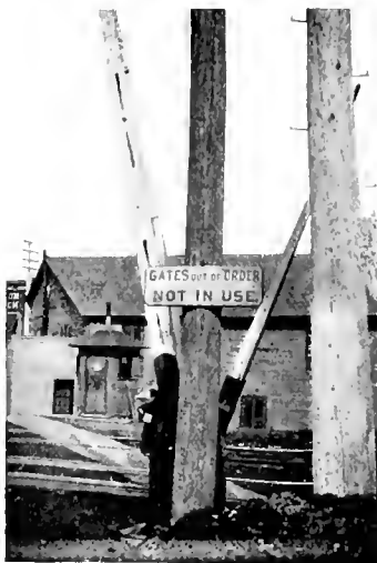
AND THESE ARE CALLED SAFETY GATES.
